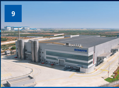
SCHÜTZ Container Systems Pvt. Ltd. INDIA – DAHEJ
